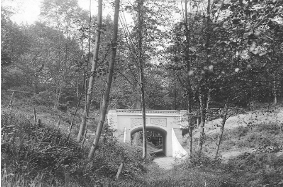
Figure 3-9: Frink Park Bridge under construction (Seattle Municipal Archives Photographic Collection - No. 29052), circa 1911
