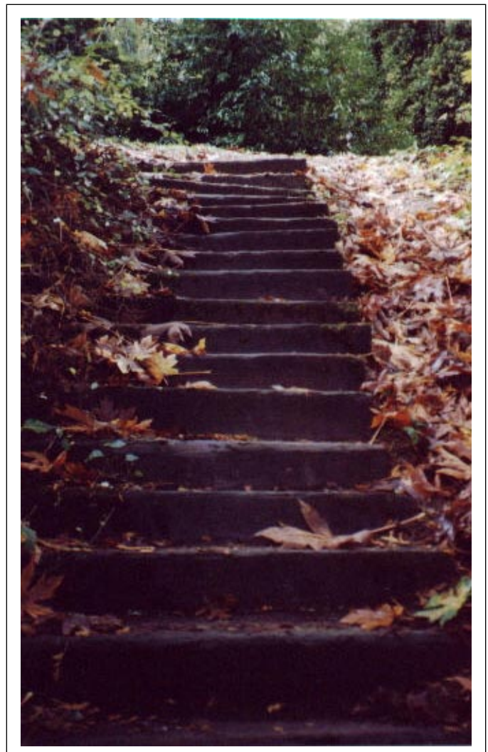
Figure 5-4. Uneven steps at ST4
