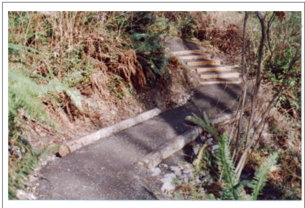
Figure 5-8. Newly constructed water crossing and stairs in Focus Area 4 demonstrate initial implementation of DPR trail standards
