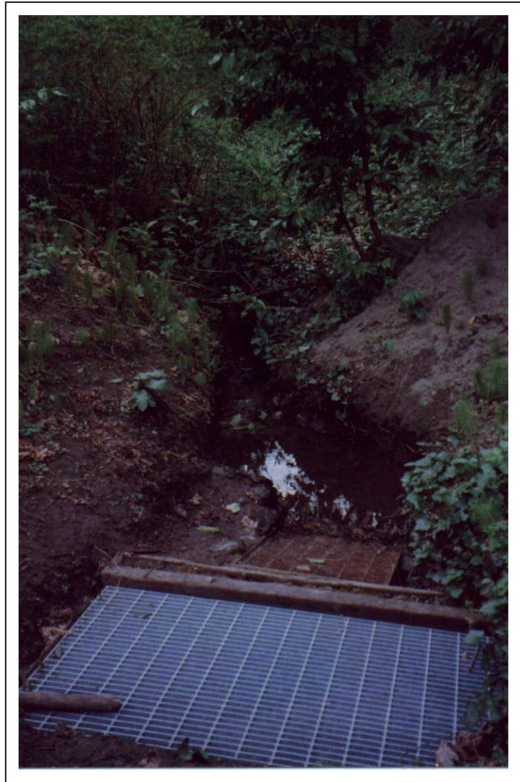
Figure 6-3. View of the catch basin and sediment pile at the stream intake
