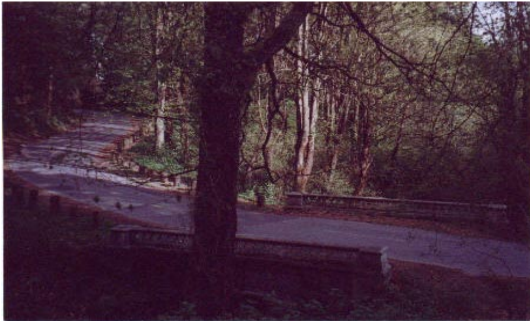
Lake Washington Boulevard, Frink Park, Seattle Washington Sheldon & Associates, Inc.
