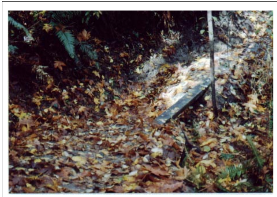
Figure 5-7. Trail erosion at water crossing prior to repairs at Focus Area 4
